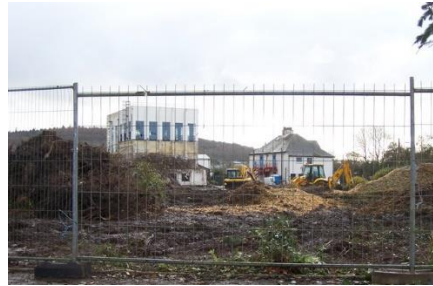
Demolition of buildings in 2012
